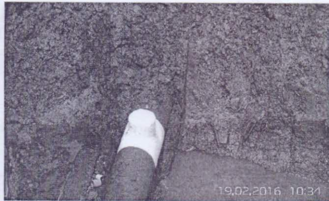
Figure 2: Conning and wrapping of the Valve
